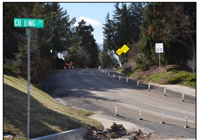
Figure 3-2. Delineated pedestrian path on Lower Braemere Road
