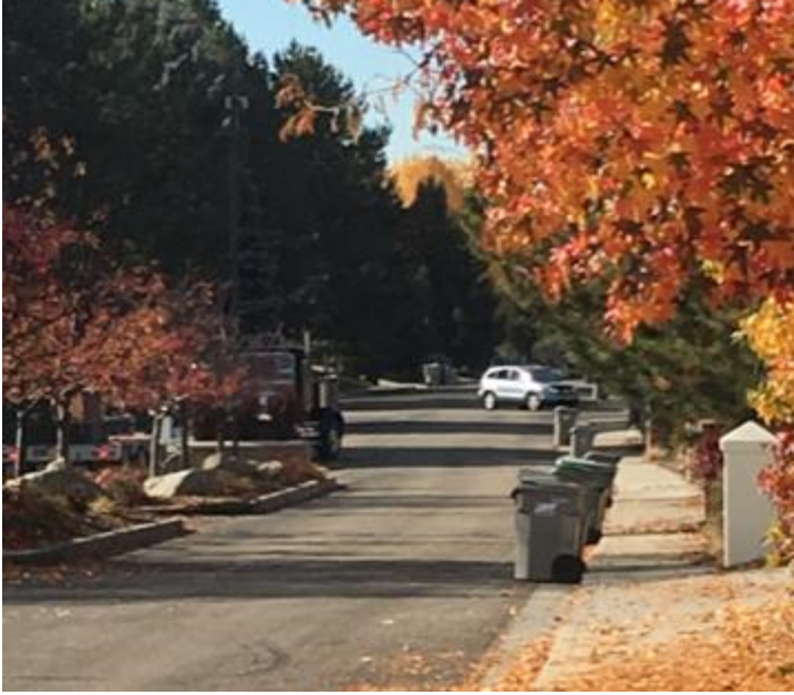
Photo 1: E. Braemere Diverter looking South – Construction traffic going the wrong way & car changing paths to avoid wrong way traffic (Date: Oct 27, 2017).
